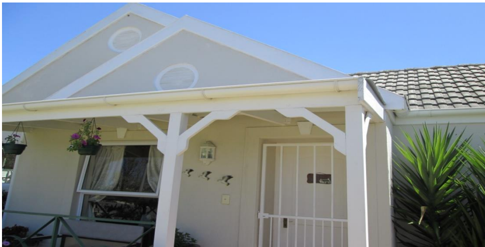
Figure D1 Configuration of décor pieces to be used with posts supporting roof structures
