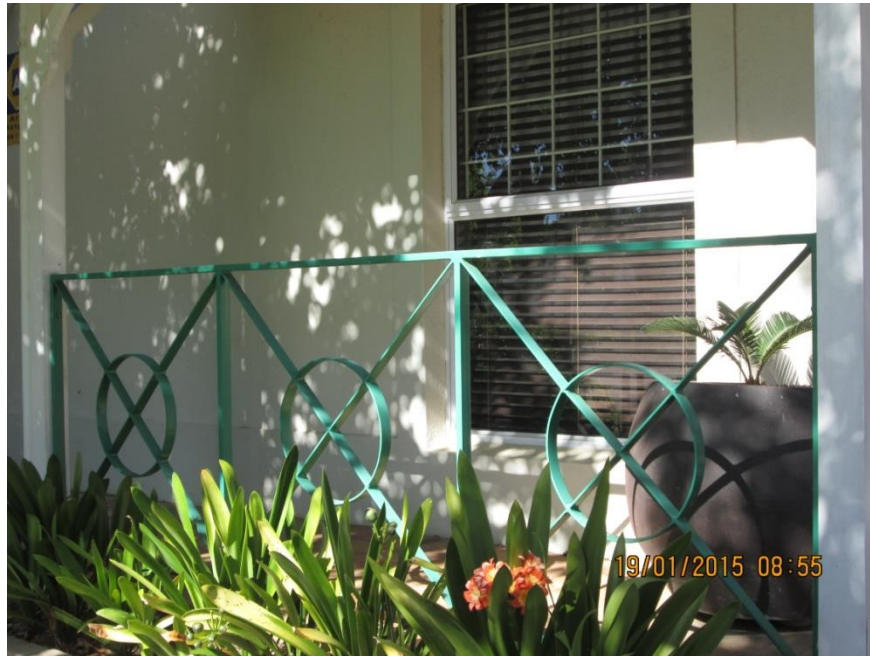
Figure C1 Permissible design of balustrades
